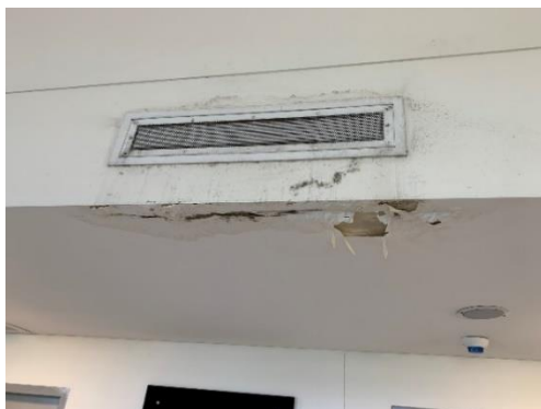
Photo 2 & 3: Water damage and mould from leaking air-conditioning units, Hume compound
