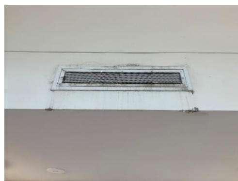
Photo 2 & 3: Water damage and mould from leaking air-conditioning units, Hume compound
