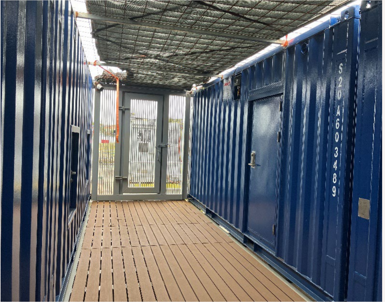
Figure 9: Enclosed walkway between accommodation modules
