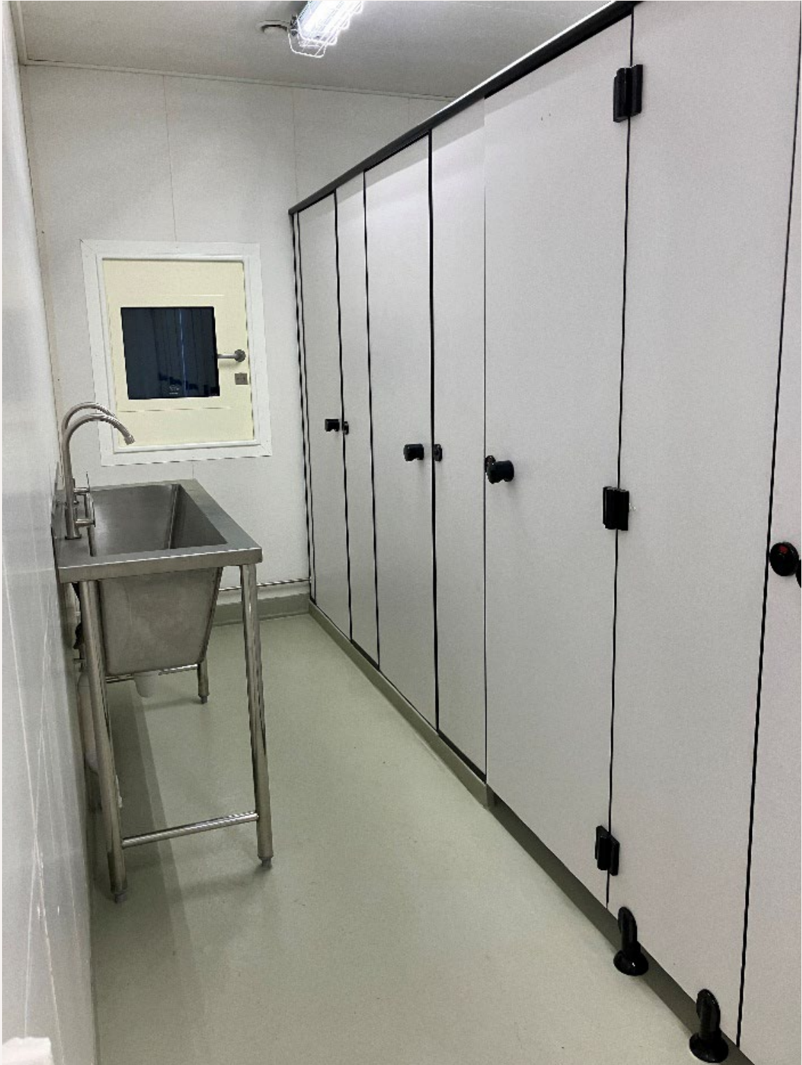
Figure 6: Interior of Ablution Module
